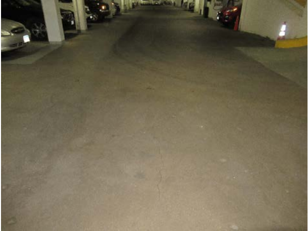
On-grade concrete garage overview
