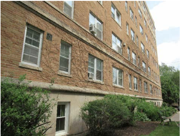
Overview of masonry with organic growth evident
