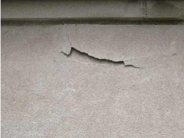
Spalled concrete
