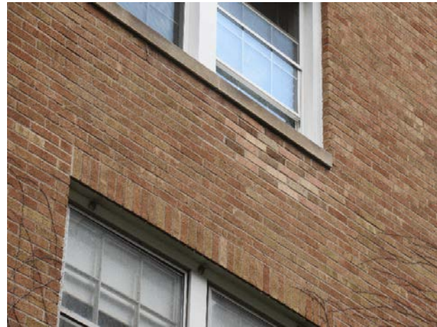
Prior masonry repairs
