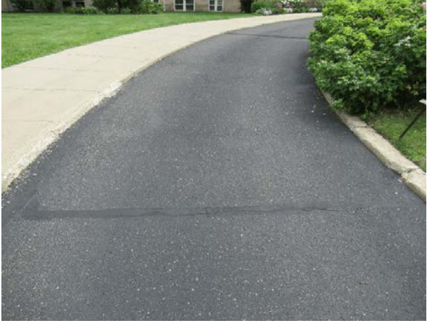
Asphalt pavement access drive overview
