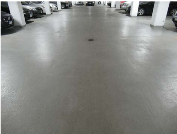
Overview of elevated concrete
