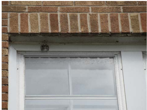
Lintel corrosion
