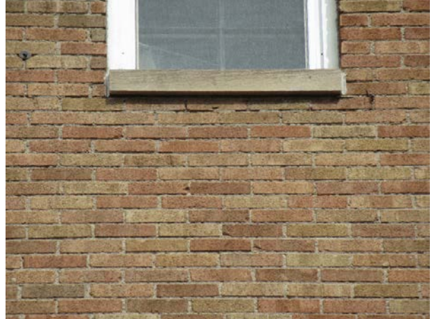
Mortar deterioration
