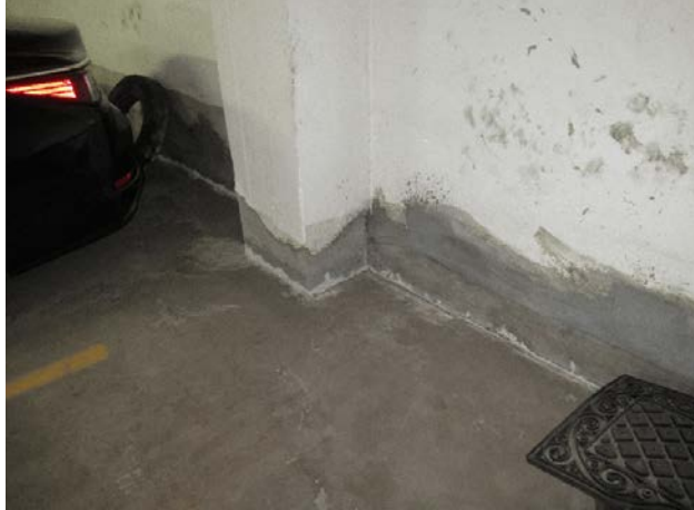
Prior wall repairs
