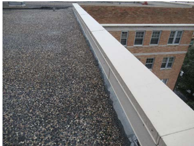
Overview of parapet wall
