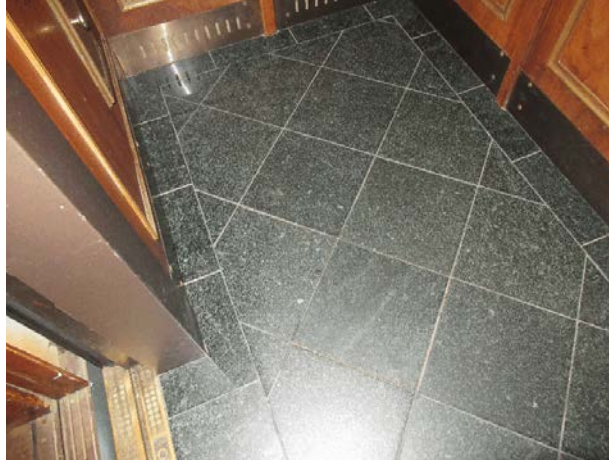
Tile floor coverings
