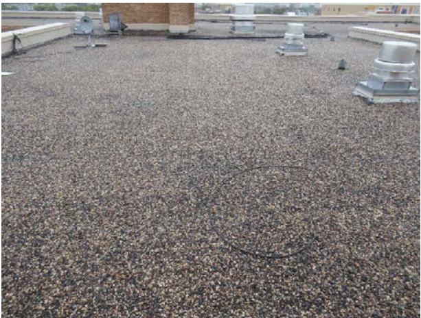
Overview of built-up roof
