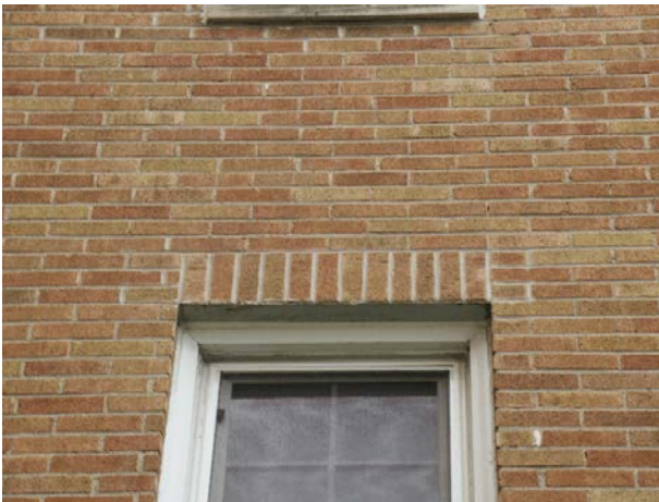
Prior repairs above lintel
