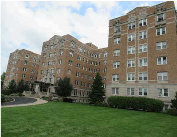
Overview of building's west elevation
