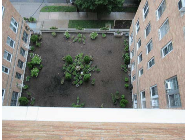
Built up roof above elevated garage
