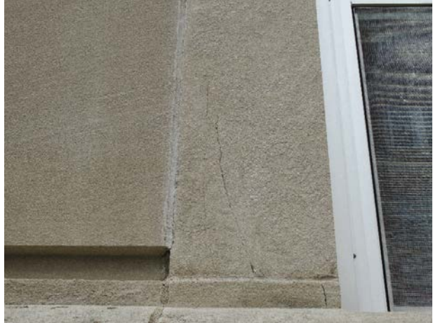
Concrete crack
