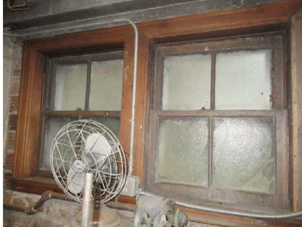
Interior view of window
