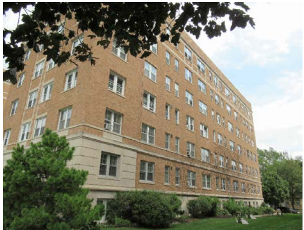
Overview of building's south elevation
