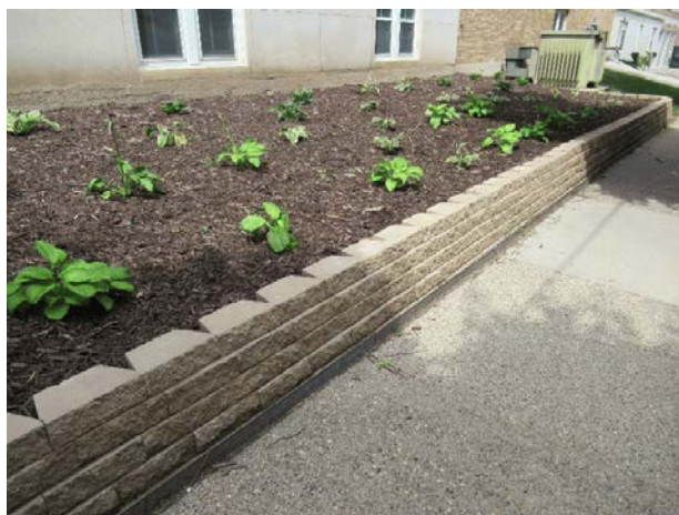
Retaining wall overview
