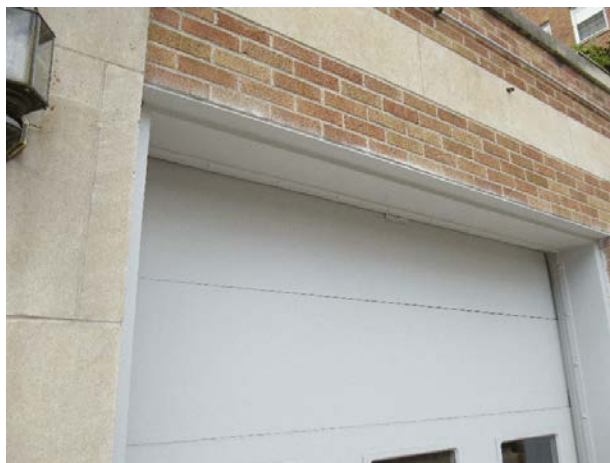
Garage lintels in good condition
