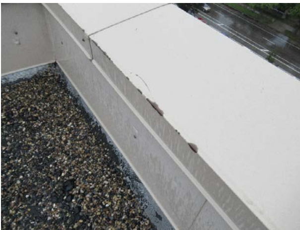
Finish deterioration
