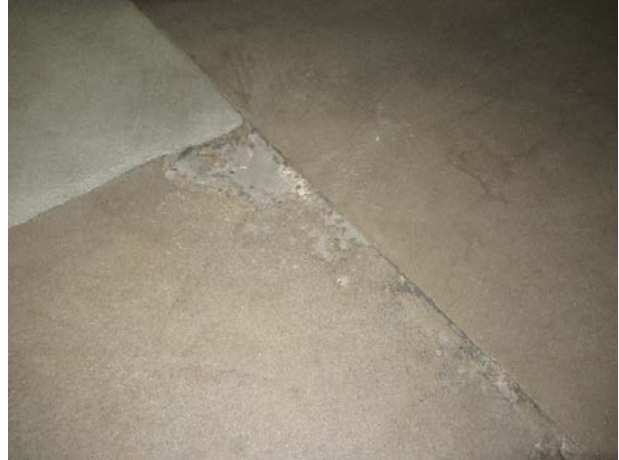
Concrete spalling
