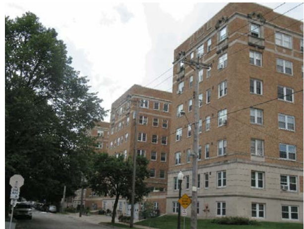
Overview of building's east elevation
