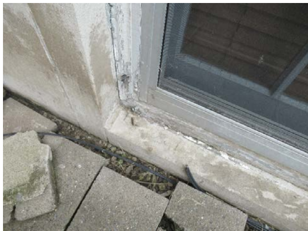
Frame deterioration
