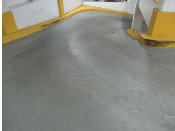
Traffic coating at ramp to on-grade parking
