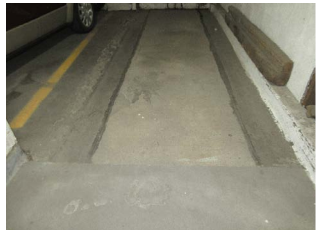
Prior slab repair
