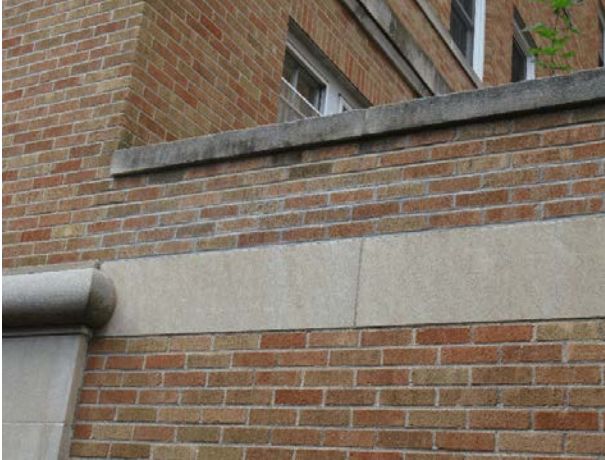
Prior masonry repairs
