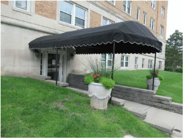
Overview of awning at north elevation
