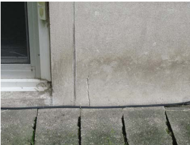
Concrete crack
